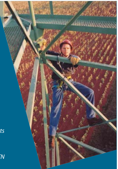
Field engineer servicing antenna support structure.
